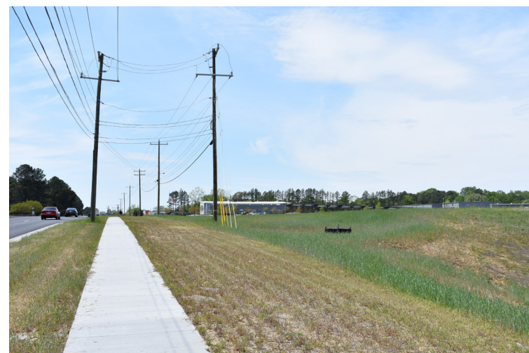
Existing view looking west
